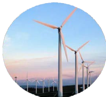
45 MW Balkhash Wind Power Station
