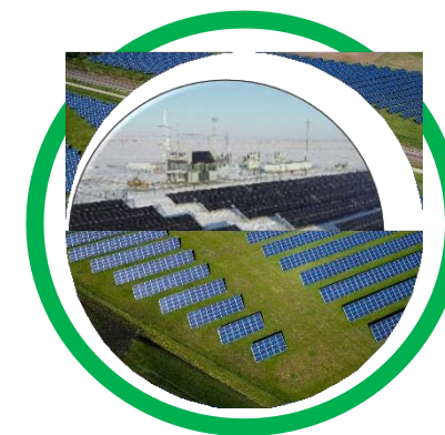
100 MW Solar Power Plant (Phase 2 – 50MW) "Balkhash"
