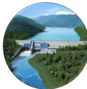
27.4 MW Hydroelectric Power Plant in East- Kazakhstan region
