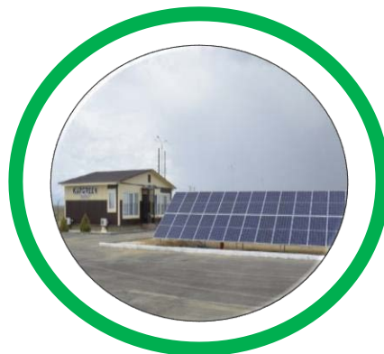
“Kengir” 10MW Solar Power Plant
