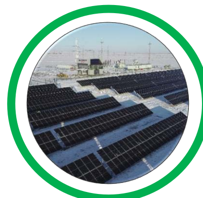
100 MW Solar Power Plant (Phase 1 – 50MW) “Balkhash”
